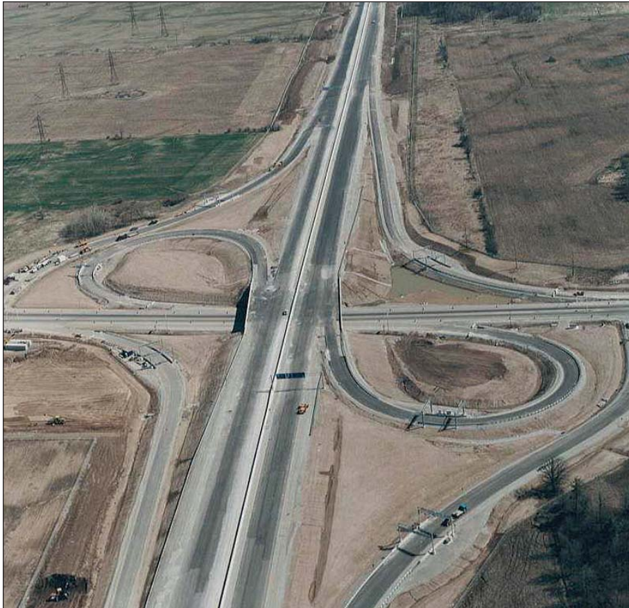
• Aerial view shows the 407 Trafalgar interchange at Oakville.
