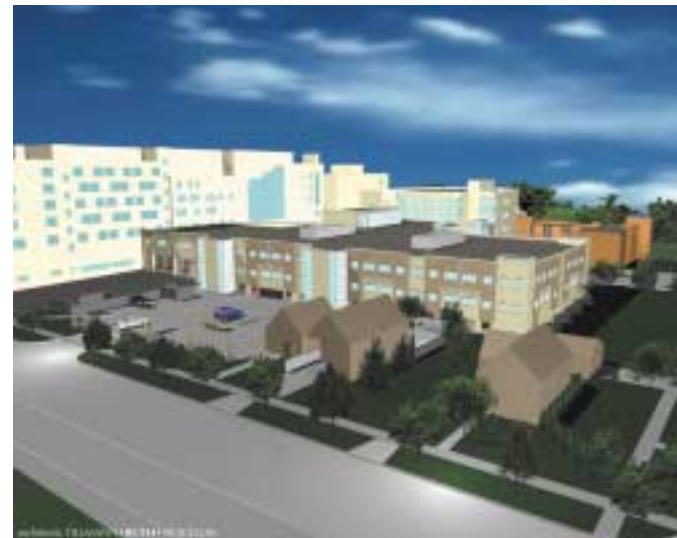
G.A. Huot Surgical Centre and Diagnostic Imaging Centre, St. Joseph's Hospital St. Joseph's Health Care, London Construction Complete 2005
