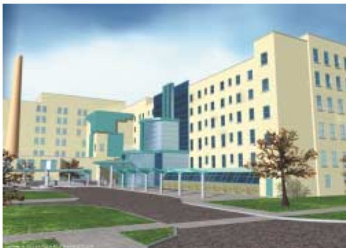
St. Joseph's Hospital St. Joseph's Health Care, London Renovation Complete 2008
