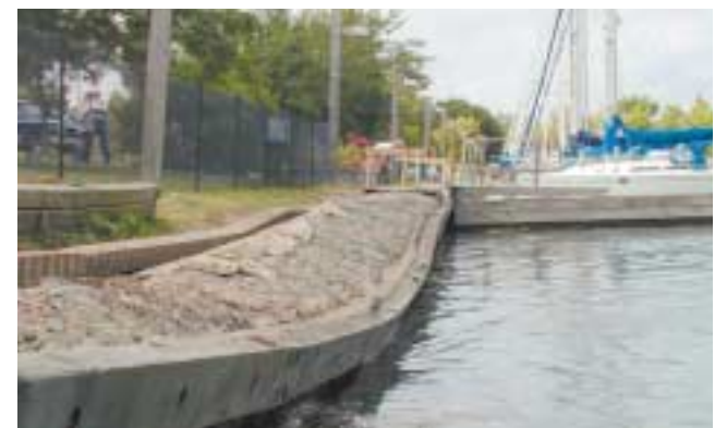
Project will repair deteriorating marina wall at Fifty Point.
