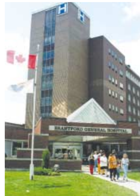
Brantford General Hospital has been serving the community since 1885.
